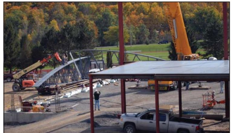
**WIDE LOAD COMING THROUGH** - The first of the steel roof supports arrived on the Utica Campus this week for the Jorgansen Athletic Center. The steel supports seen on the truck to the left are half of the span of the roof. These sections are attached and then hoisted by a very large crane. As of Friday, there were five roof supports in place. Other work completed this week includes a cinder block wall for one side of where the athletic surface will be.
